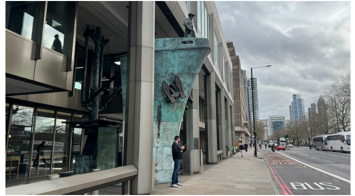
IMO Building, Albert Embankment, London
