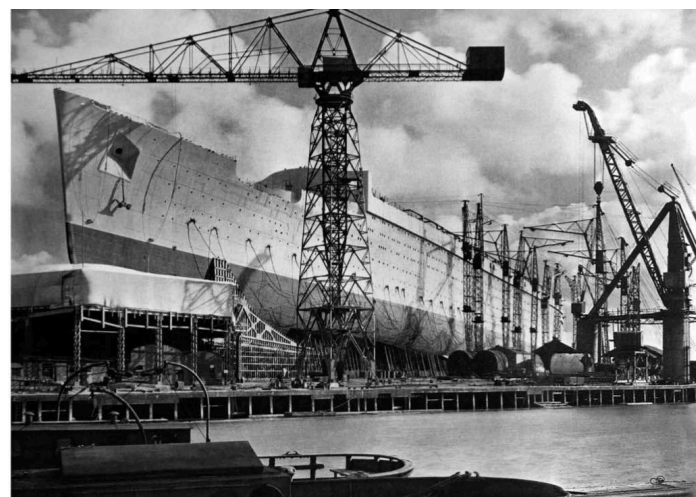
Almost ready for launching with much of the scaffolding removed.
